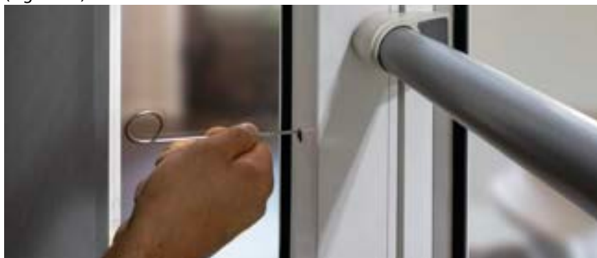
Figure 11: Inside access to emergency opening
